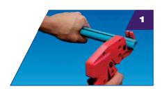
Ensure the pipe is cut square and cleanly, using approved 'ratchet style' pipe cutters on the 25 and 32mm and using a fine tooth saw or wheeled cutter on the 63mm.
