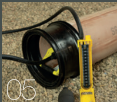
05 Allow approx. 5 minutes for stabilisation before adjusting the pressure to 100mm water gauge.
