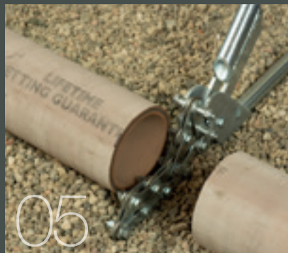
05 Push down on the handle to snap cut the pipe
