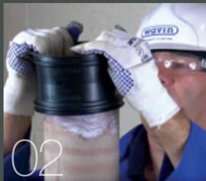
Press the coupling on to the lubricated pipe end
