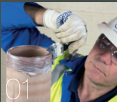
Lubricate the pipe end
