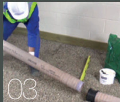
Push into previously laid SuperSleve pipe
