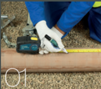
01 Mark the pipe to be cut
