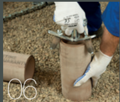
06 Remove any sharp edges with pipe trimmer
