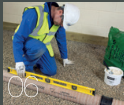
Check the pipeline is laid to the correct gradient
